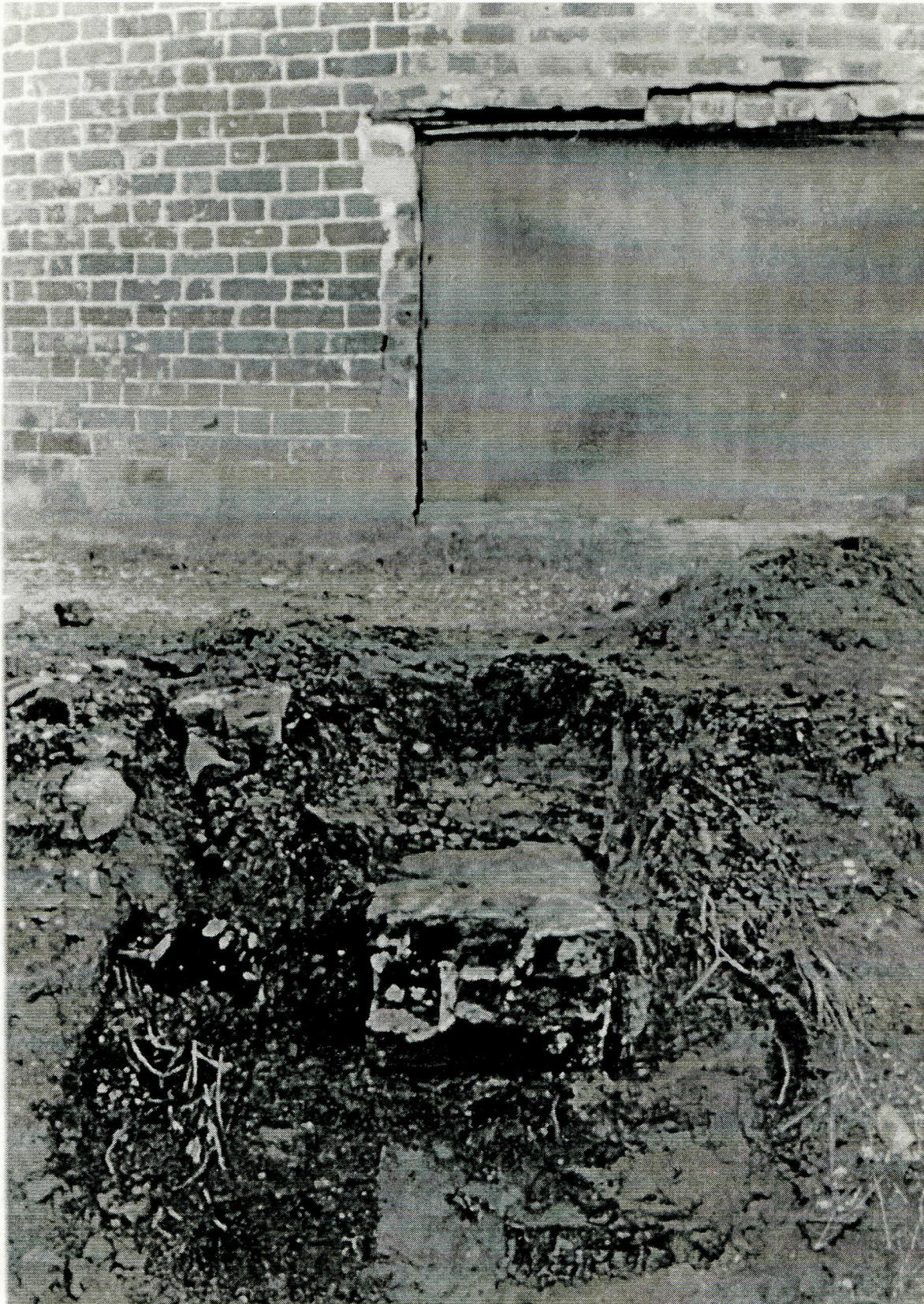
Figure 9 Photograph of the foundation steps, 1987
